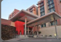
Rosebank development completed
