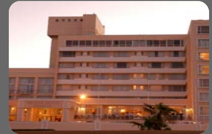
Protea Hotel Marine refurbished
